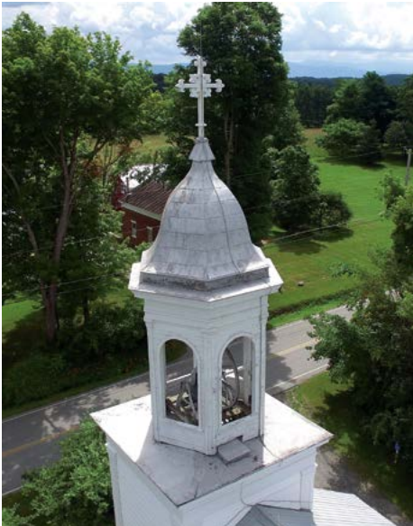
CRM Associates drone photo-inspection of Charlotte church bell tower.
